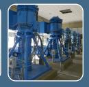
is treated with ozone to kill organisms and break down contaminants. Ozone is produced on-site from air, bubbled into the water, and then converted back into oxygen.
