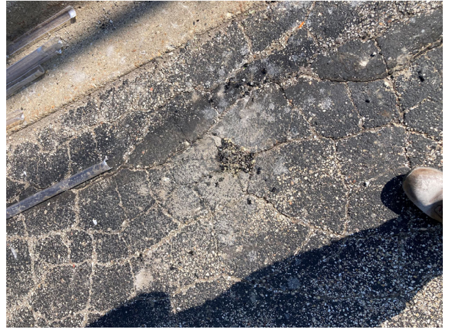
#8: View of SB-4 backfilled to grade with bentonite and asphalt patching.
