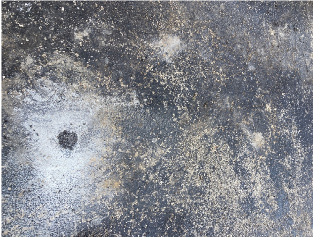
#7: View of SB-3/TW-3 backfilled to grade with bentonite and asphalt patching.
